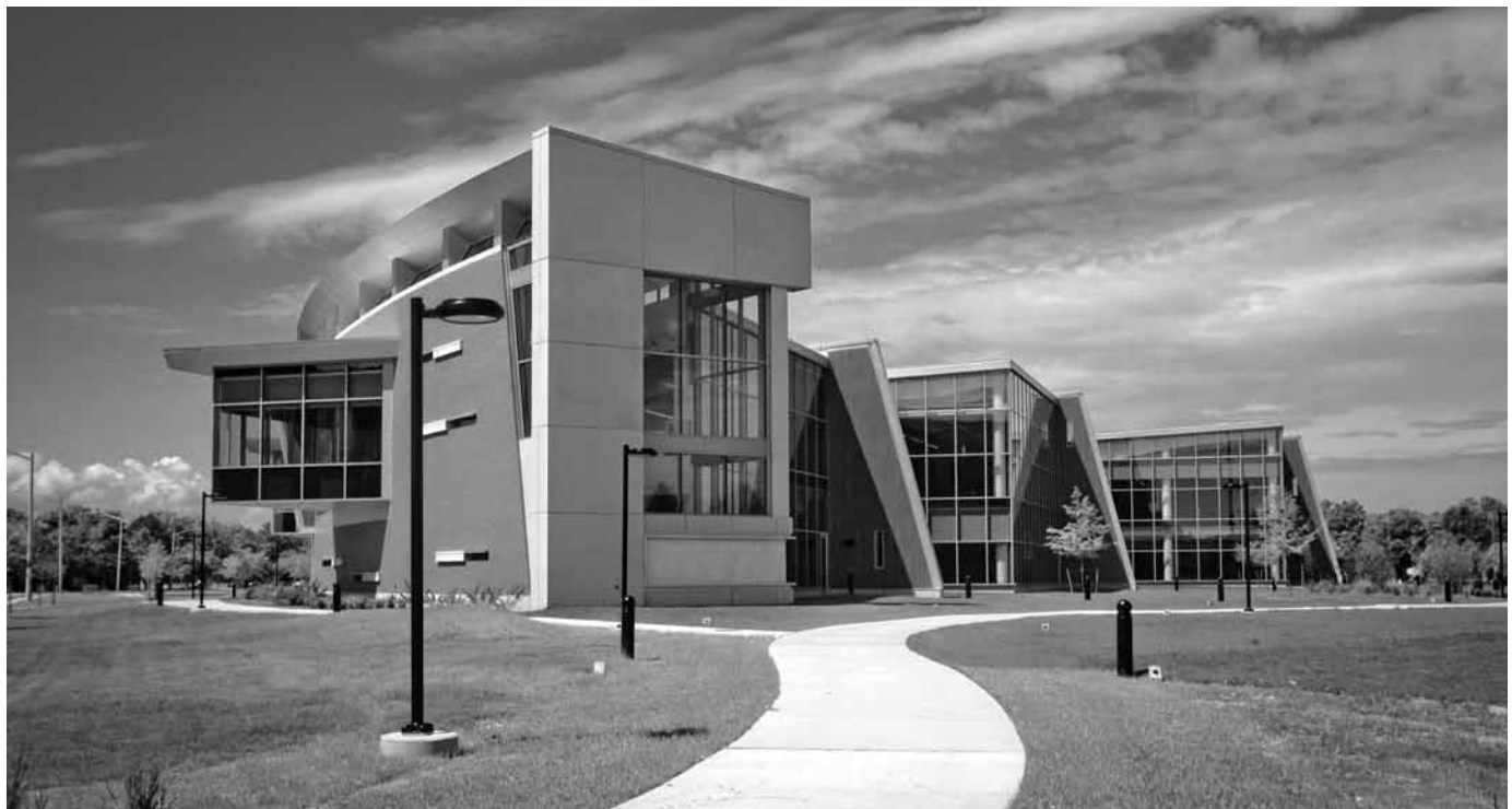
The new $43 million, 125,000-square-foot joint-use library serves the needs of both Virginia Beach and Tidewater Community College.
