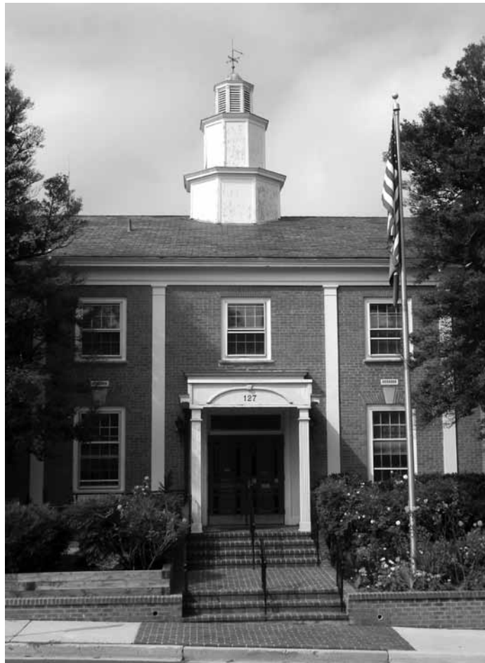
Vienna Town Hall's renovation took about 10 months to complete.
